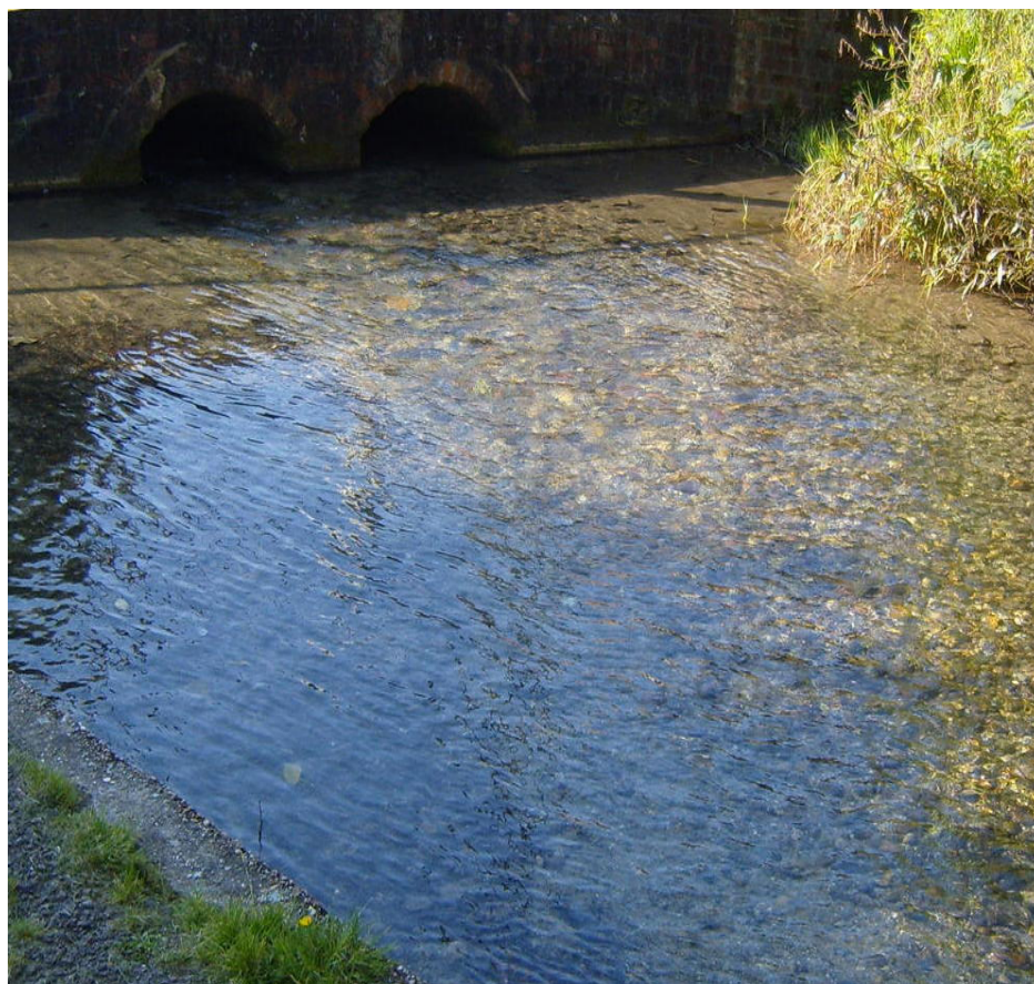
Figure 2 (b): the stream at Kingsclere.
